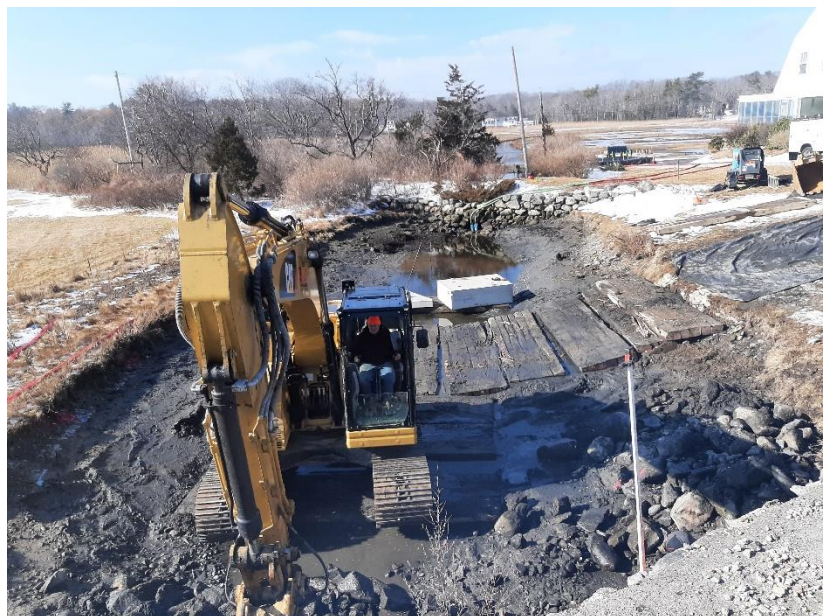
Removal of the stone weir in early 2022. Photo credit: Frank Arcidiacono, North Hampton Conservation Commission.
