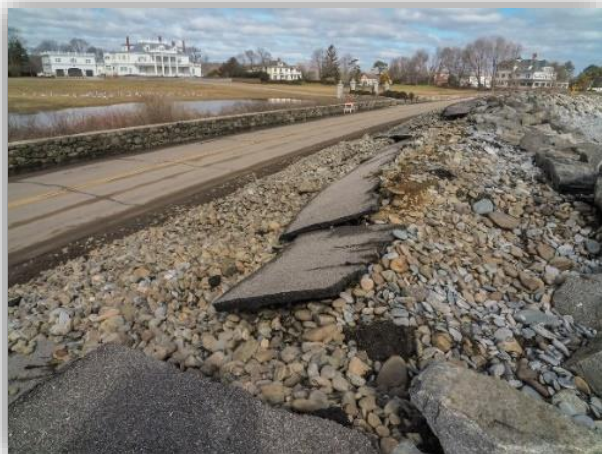
Broken walkway along the Route 1A shale piles after a coastal storm in March 2018. Photo credit: Rich Beauchesne.
