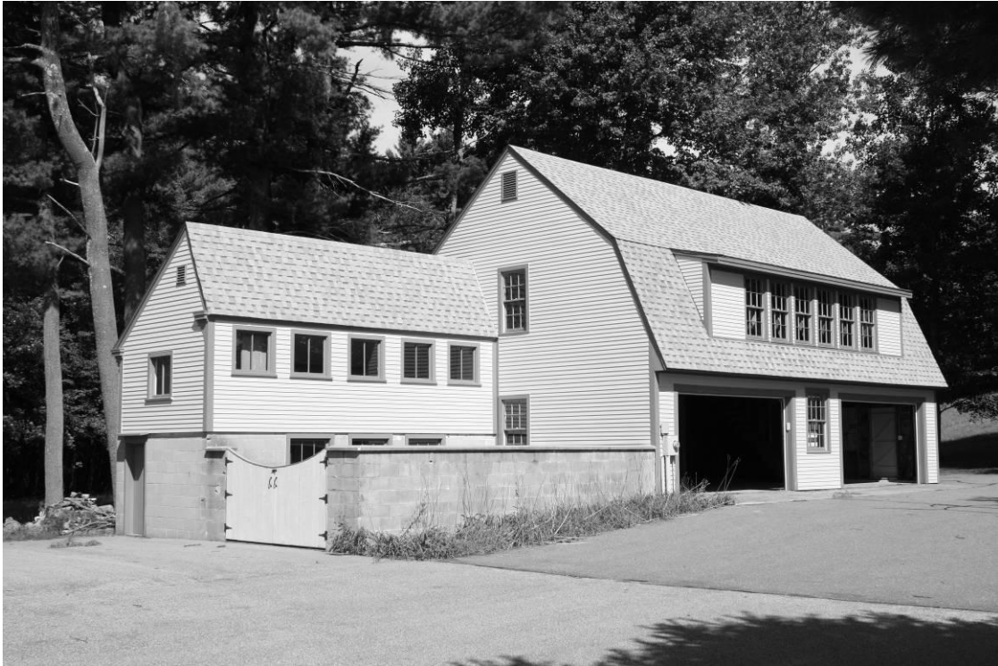
Photo # __14__ Description: South and east (façade) elevations of poultry barn/pig pen Digital file name: NHA0010_14 Direction: NW
