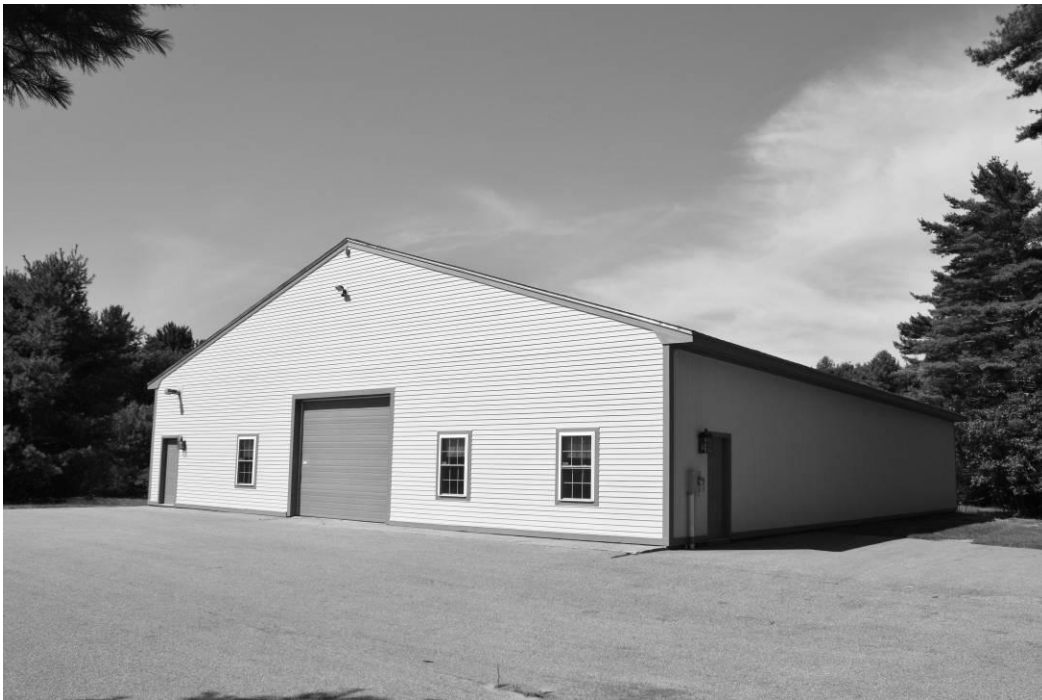
Photo # __17__ Description: Storage building, east (façade) and north elevations Digital file name: NHA0010_17 Direction: SW
