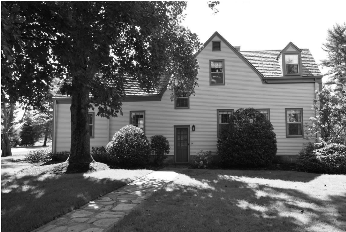
Photo # __8__ Description: North elevation of main house Digital file name: NHA0010_8
