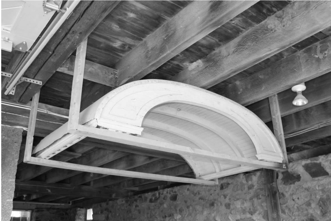
Photo # 6 Description: Original entrance porch roof, stored in lower level of barn Digital file name: NHA0010_6 Direction: NE
