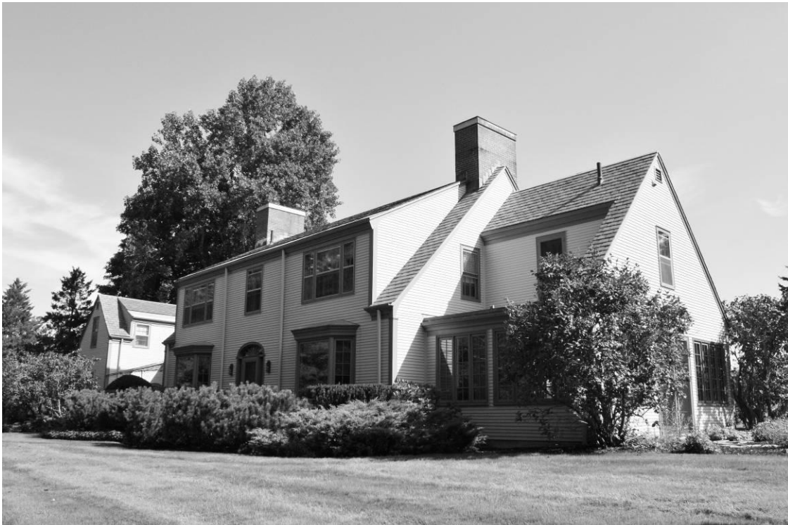
Photo # 7 Description: West (rear) and south elevations of main house Digital file name: NHA0010_7 Direction: NE
