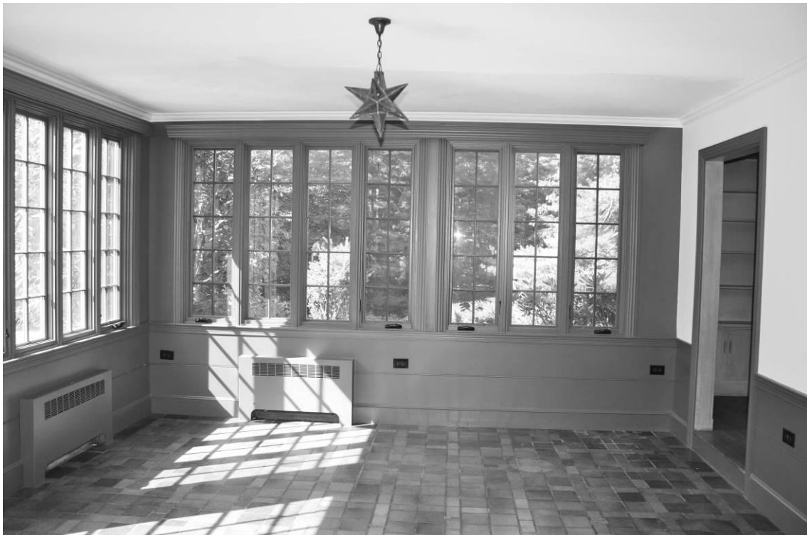
Photo # __11__ Description: Main house, first floor sunroom Digital file name: NHA0010_11 Direction: SW
