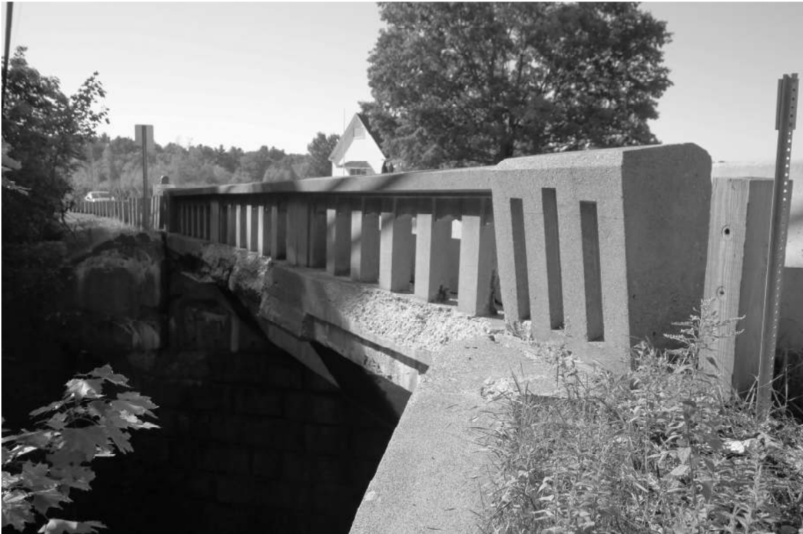
Photo 19) cast concrete railings, south side Reference (file name): NHA0002_019
