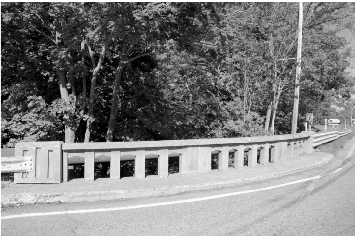
Photo 16) cast concrete railings, north side Reference (file name): NHA0002_016
