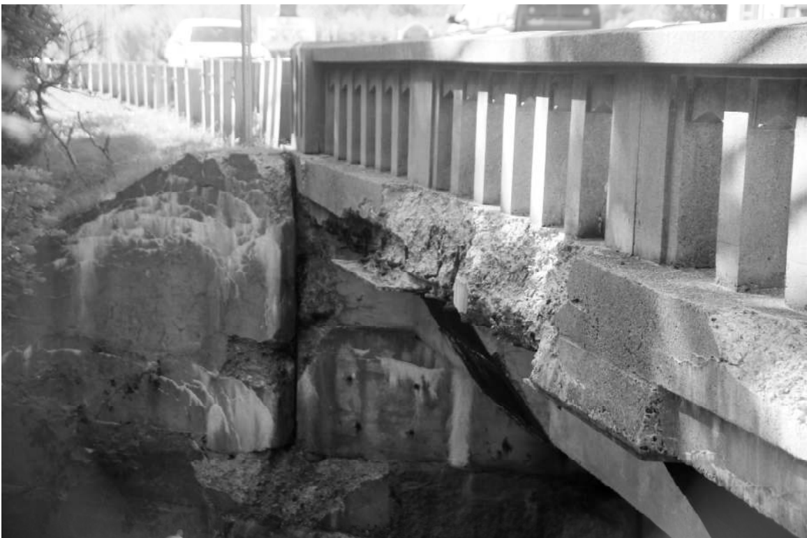
Photo 20) detail of cast concrete railing and deterioration, south side Reference (file name): NHA0002_020
