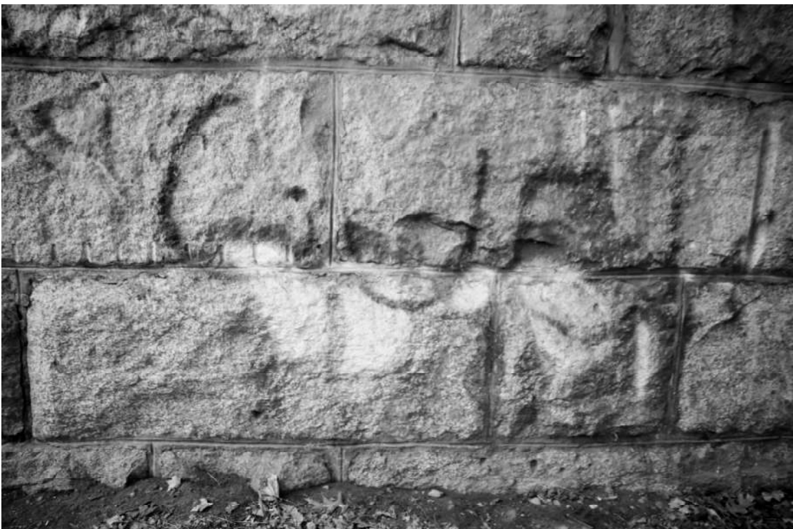
Photo 12) detail of granite blocks with graffiti and quarry marks Reference (file name): NHA0002_012
