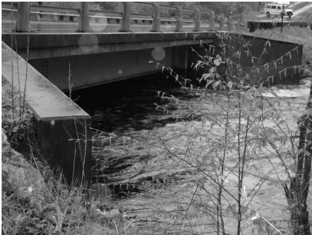
Barrington 075/122 (Note: exterior stringer apparently added 1984) (NHDOT 2006)
