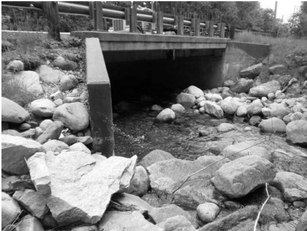
Shelburne 049/089 (Note: the east side of the bridge is CTB. On the west side the concrete beams have been replaced with I-beams) (NHDOT 2013)
