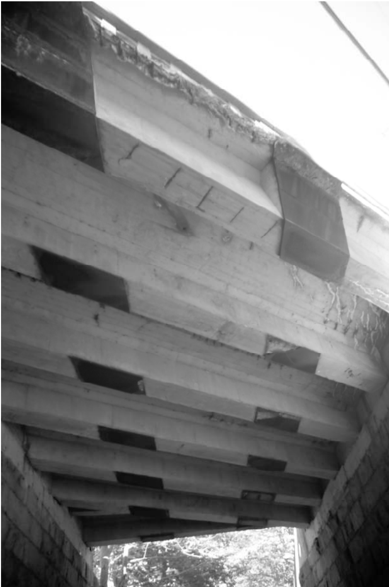
Photo 10) concrete T beams with blast plates Reference (file name): NHA0002_010
