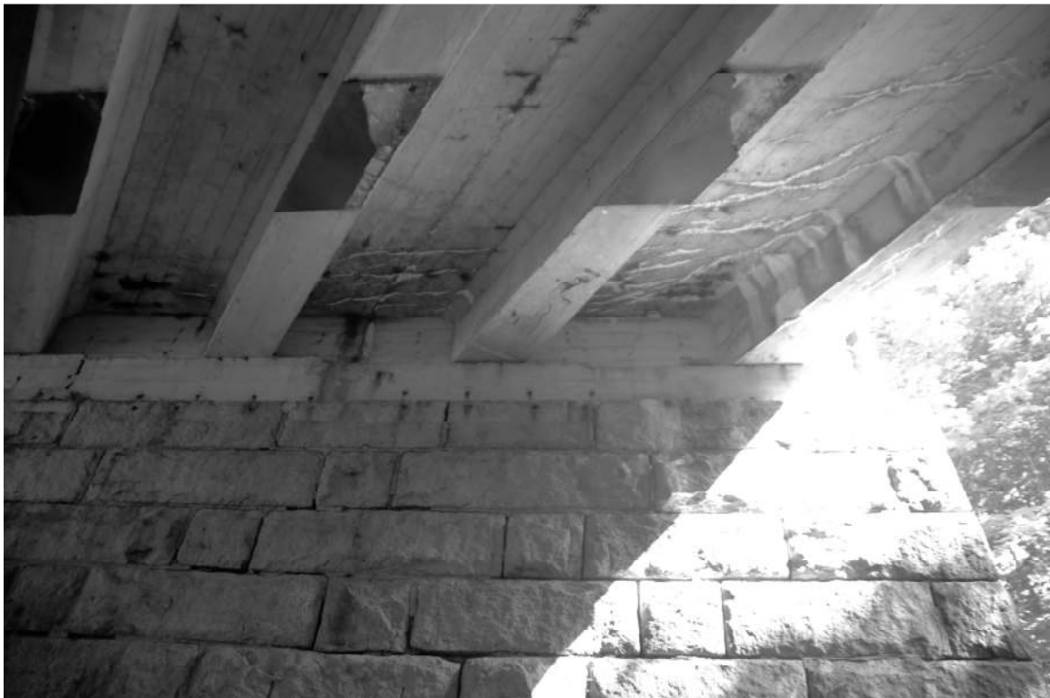
Photo 13) detail of concrete T beams and eastern wall Reference (file name): NHA0002_013
