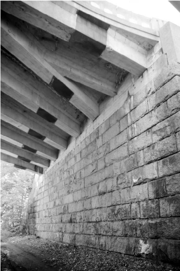
Photo 5) western substructure and concrete beams with blast plates Reference (file name): NHA0002_05
