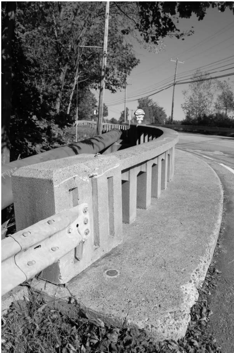
Photo 18) detail of northwest corner of cast concrete railing Reference (file name): NHA0002_018
