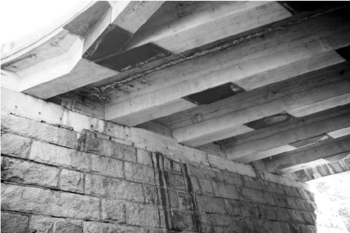
Photo 6) eastern substructure and concrete beams with blast plates Reference (file name): NHA0002_06
