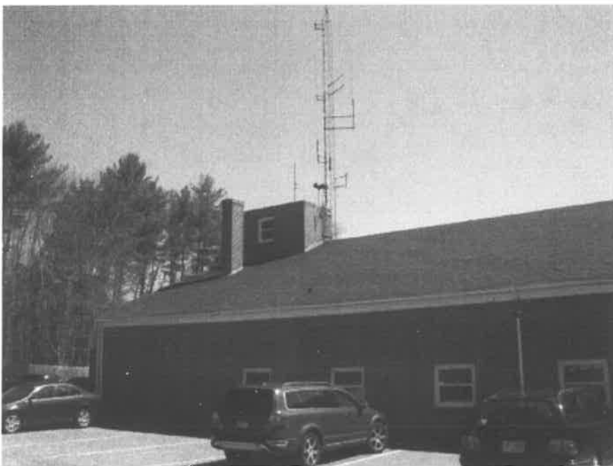
Photo 2: West Elevation, fire tower and antenna tower.
