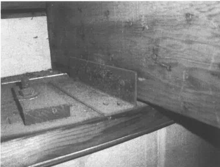
Photo 7: Truss bearing, clip angle, wall plate
