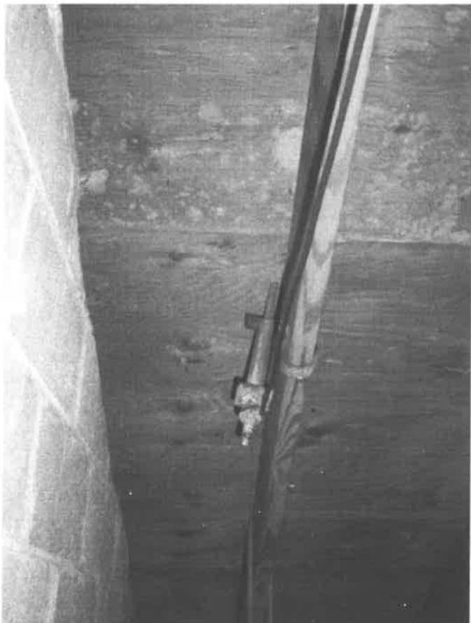
Photo 5: Antenna guy anchorage to truss top chord.
