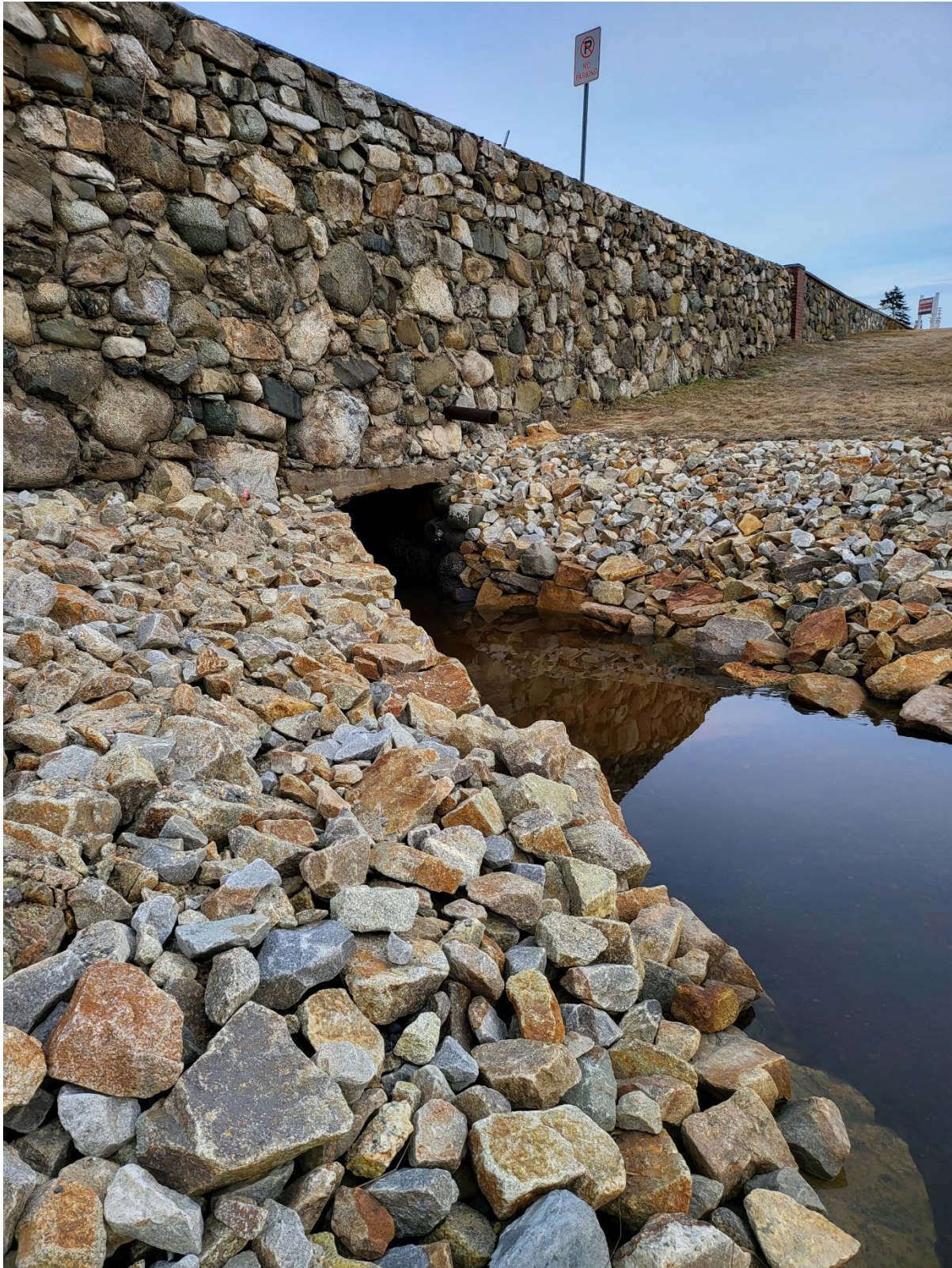
1. Philbrick Pond Culvert Inlet, March 15, 2022
