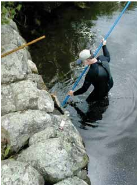
Figure 3 Testing the Trolley Berm Pipe
