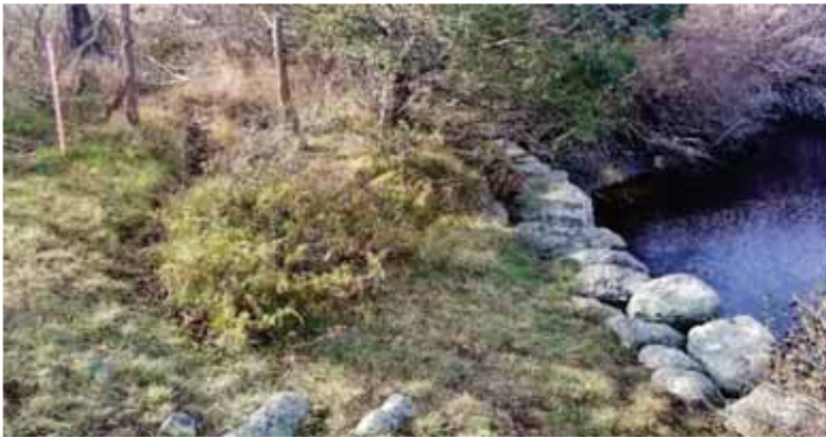
Figure 2 1900 Vintage Trolley Berm Surface
