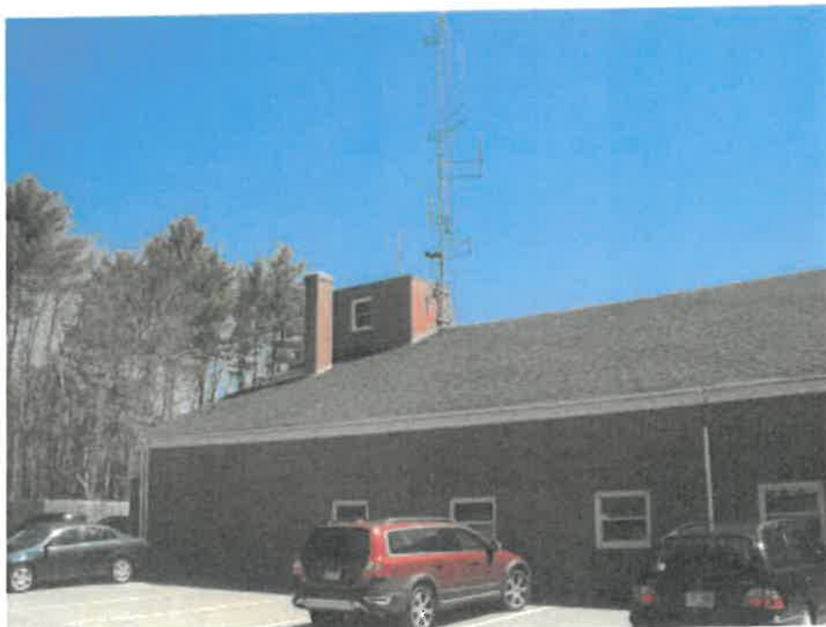
Photo 2: West Elevation, fire tower and antenna tower.
