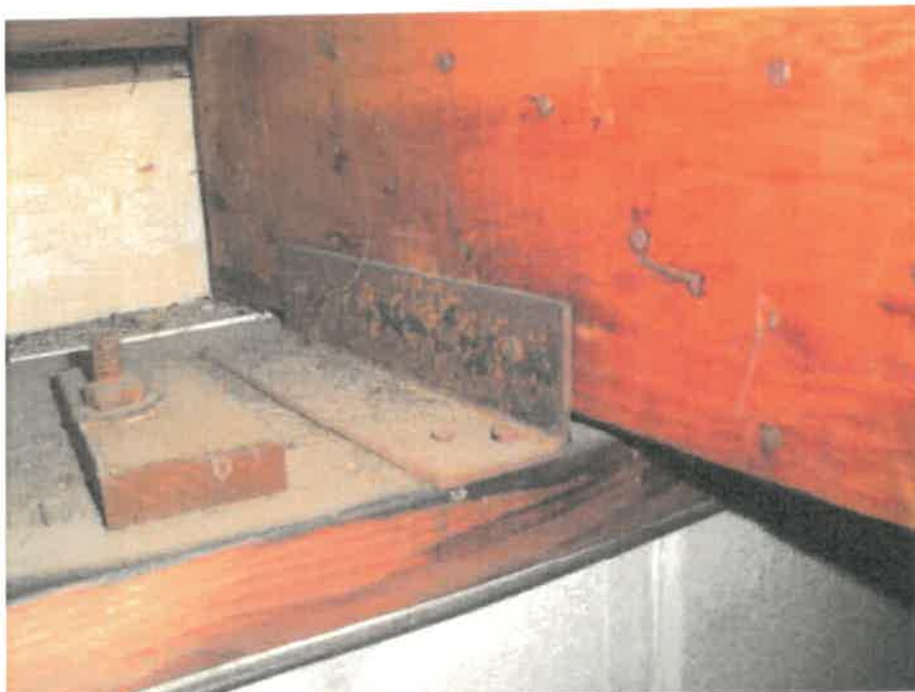
Photo 7: Truss bearing, clip angle, wall plate
