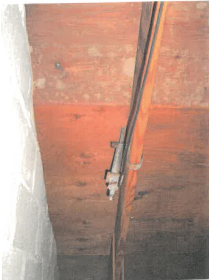
Photo 5: Antenna guy anchorage to truss top chord.
