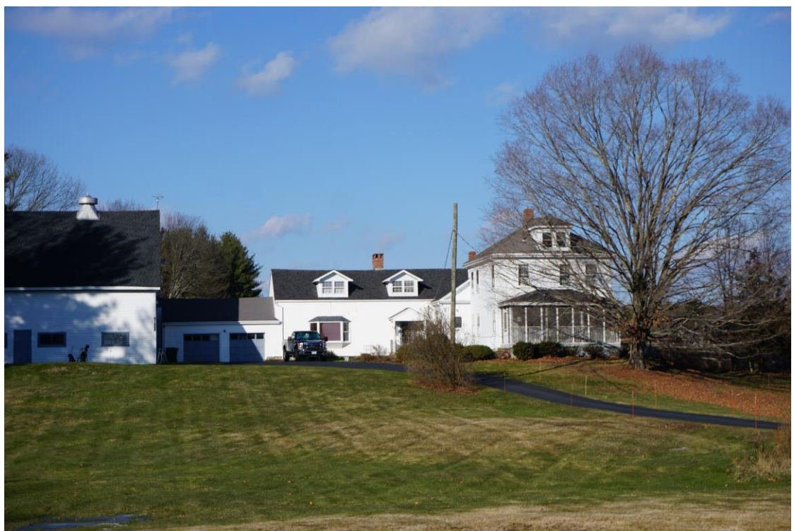
Photo # _136__ Description: 93 Exeter Road Reference: ExeterRd_93 Direction:
