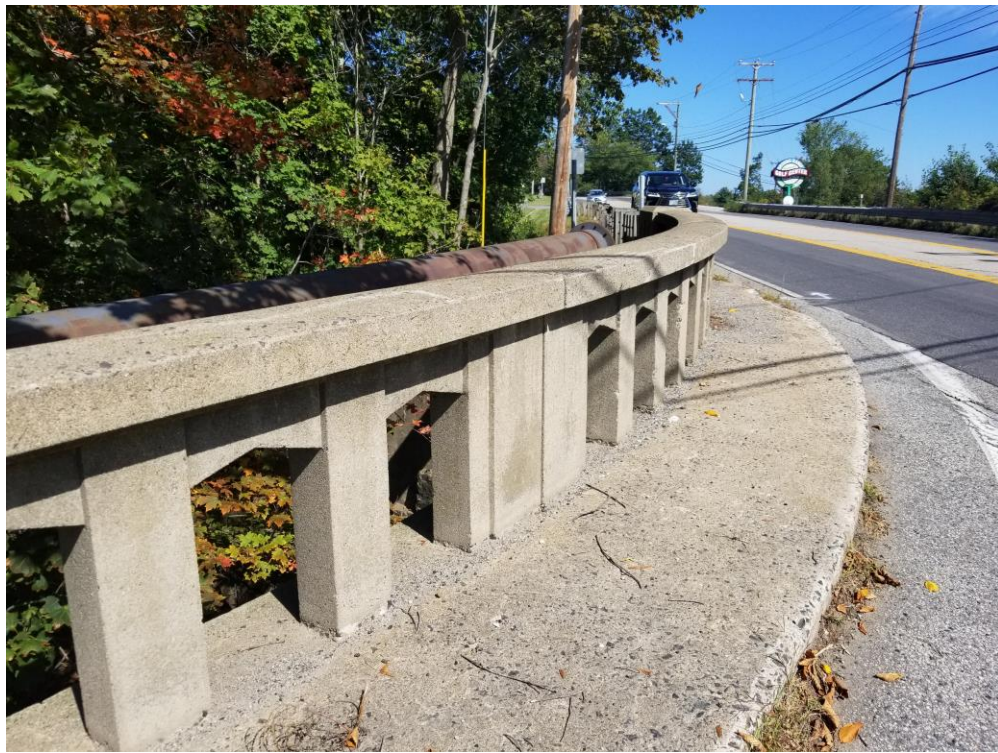
Photo # _167____ Description: Drake Bridge, Lafayette Road over RR
