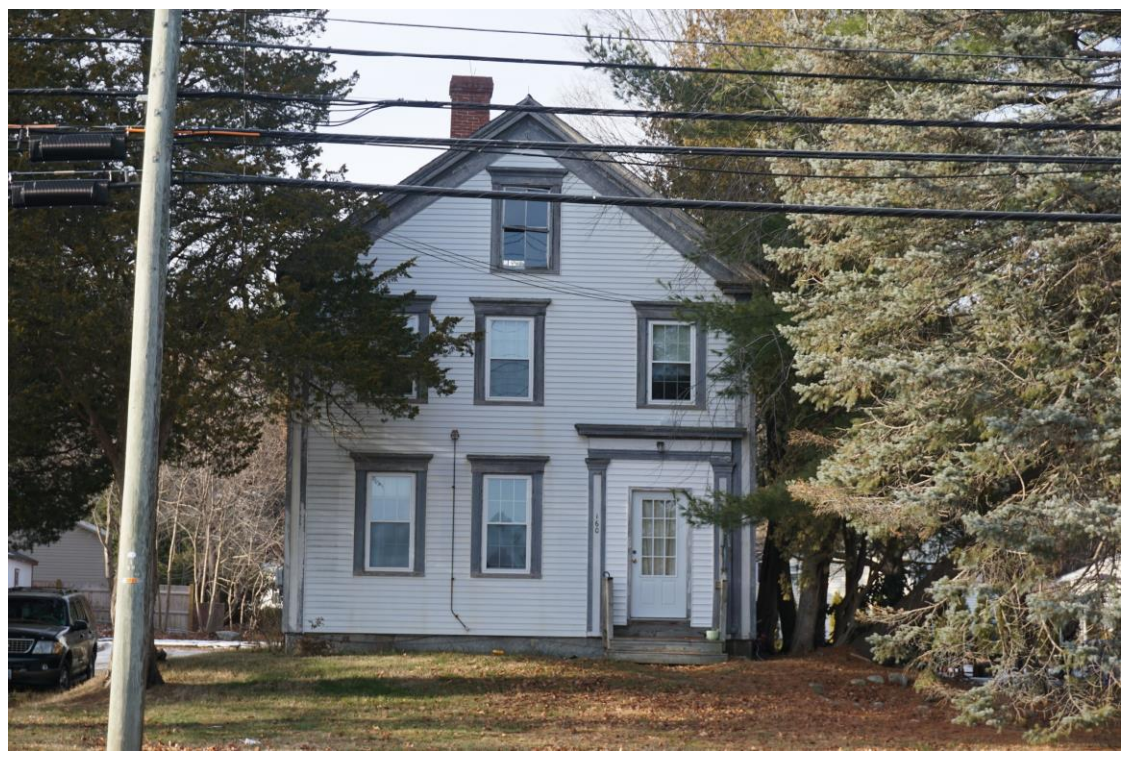
Photo # __56__ Description: 160 Lafayette Road
