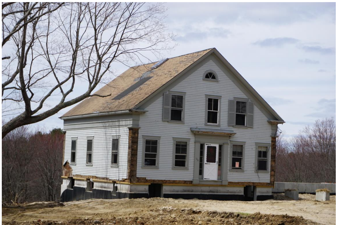
Photo # __52__ Description: 146 Post Road Reference: PostRd_146 Direction:
