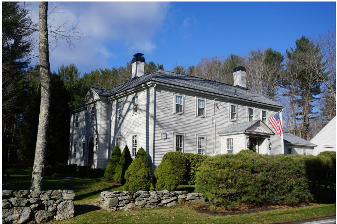
Photo # _25_ Description: 100 Mill Road
