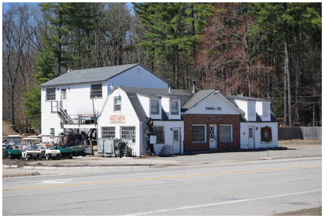
Photo # __173__ Description: 74 Lafayette Road
