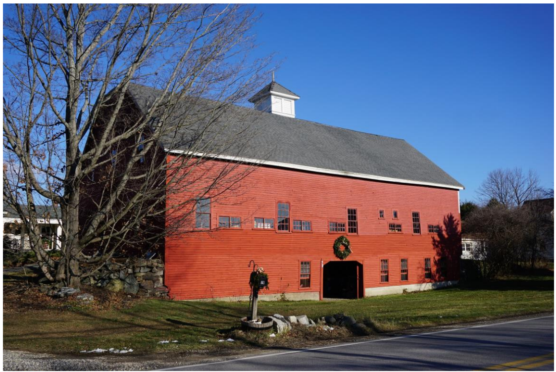
Photo # _189___ Description: Bank barn, 79 South Rd.
