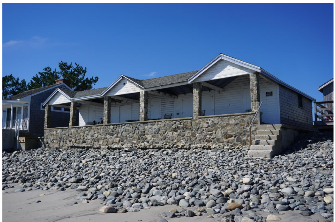
Photo # __132__ Description: Fuller Bathhouse, 17 Ocean Blvd.
