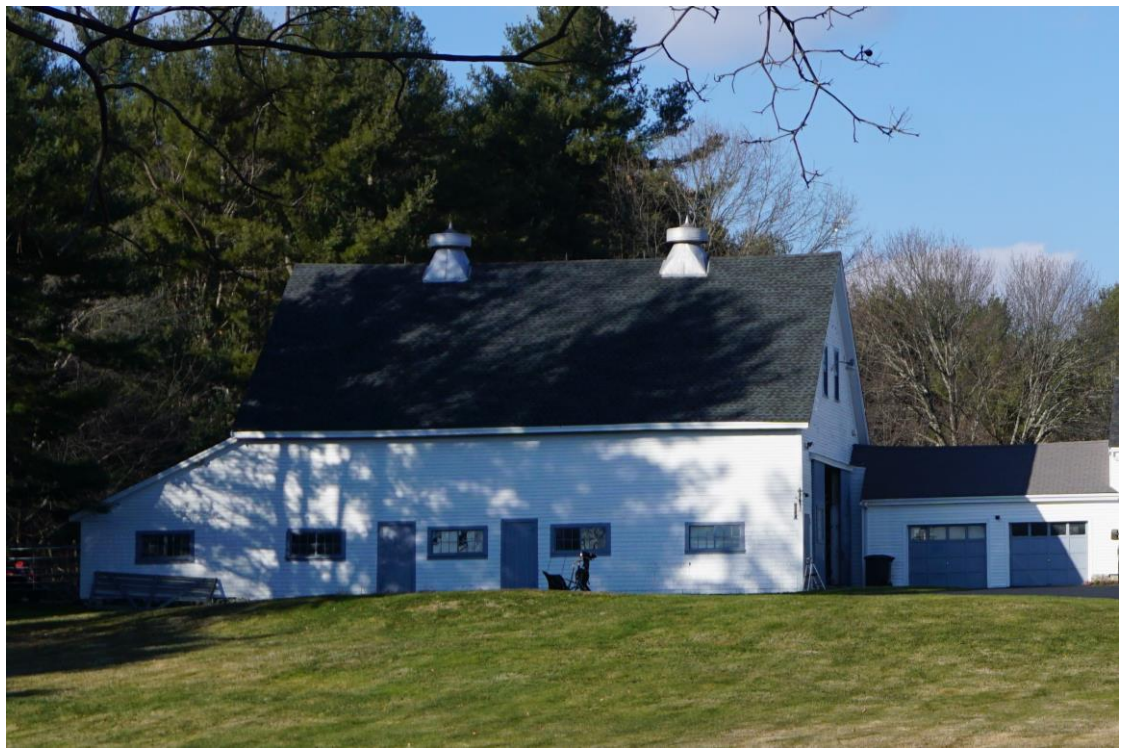
Photo # 185 Description: Barn, 93 Exeter Road
