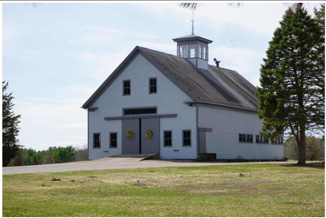
Photo # __188___ Description: Bank barn, 182 Post Road
