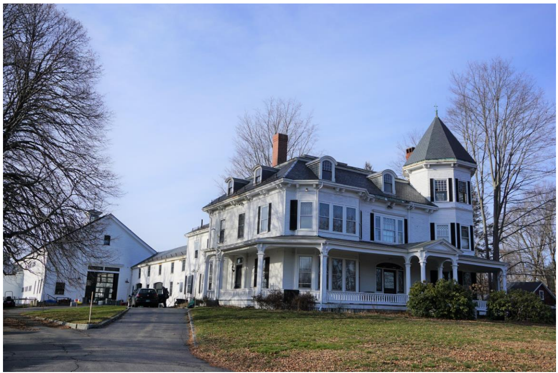
Photo # __69__ Description: 2 Elm Road
