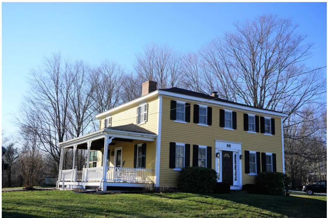
Photo # _26_ Description: 88 Post Road
