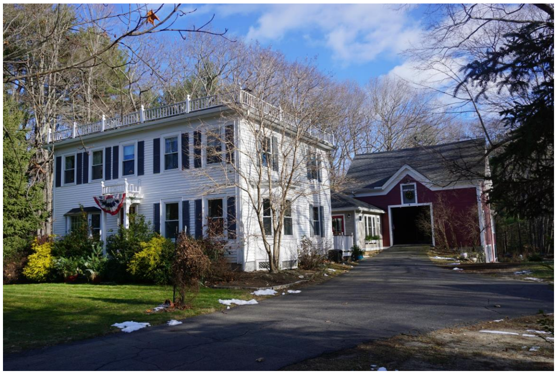
Photo # __41__ Description: 39 Pine Road
