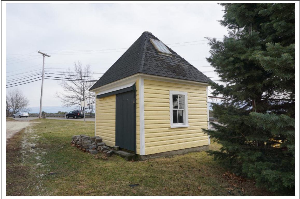
Photo # __193__ Description: Well house, 148 Lafayette Road Reference: LafayetteRd_148-2 Direction:
