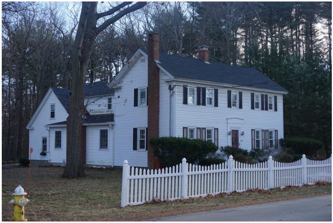
Photo # __12__ Description: 43 Pine Road
