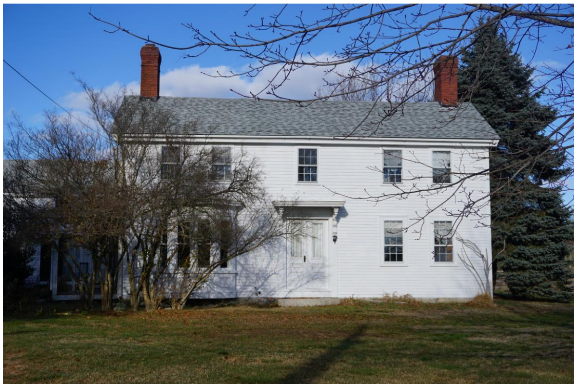
Photo # __75__ Description: 19 Maple Road
