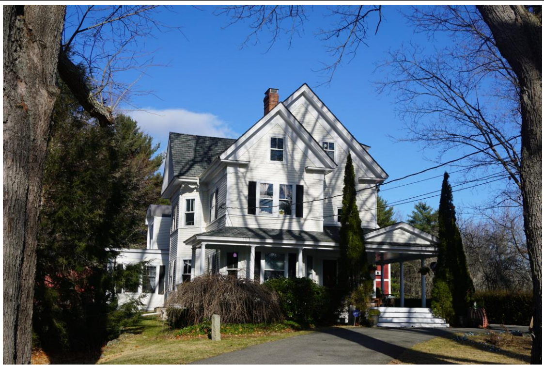
Photo # __98__ Description: 31 Maple Road
