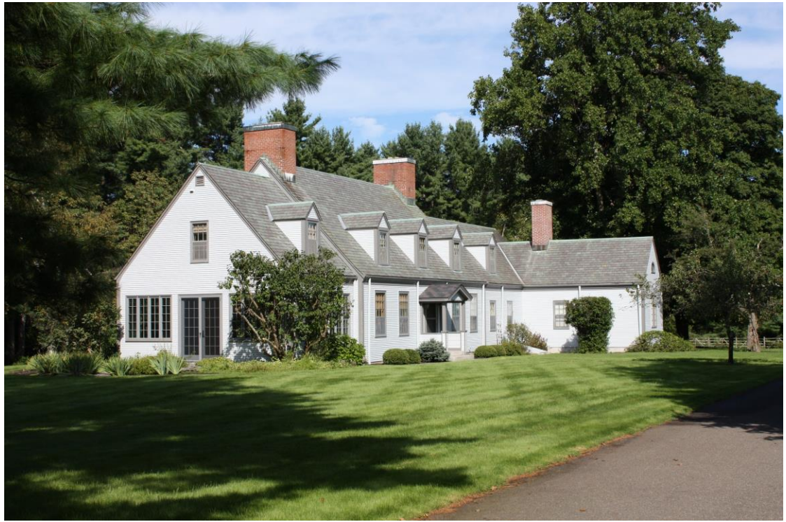
Photo # __147__ Description: Dale House, 186 Post Road Reference: PostRd_186
