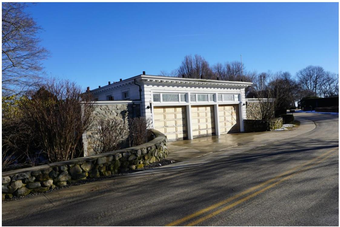
Photo # _197___ Description: Fuller Garage, 15 Willow Ave.
