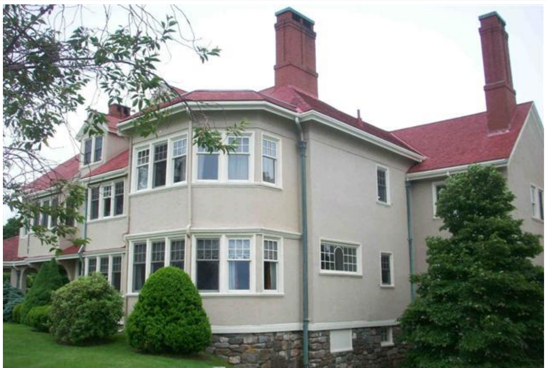
Photo # _130_ Description: 34 Willow Avenue
