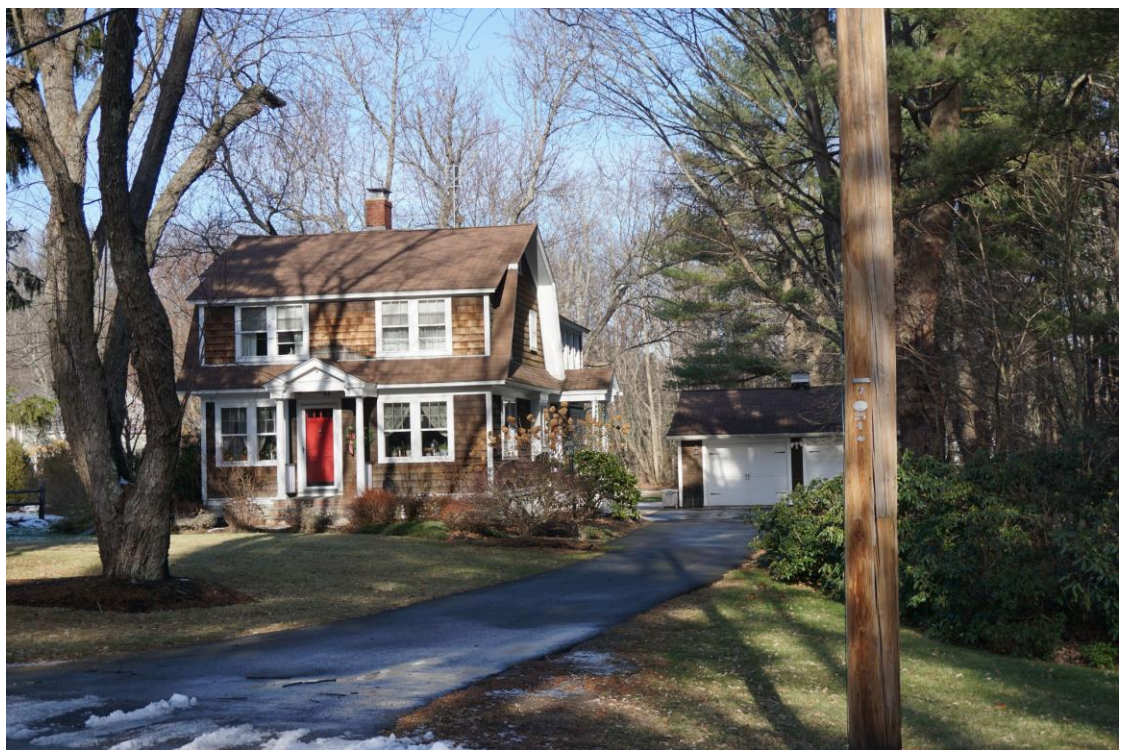
Photo # __144___ Description: 21 New Road Reference: NewRd_21 Direction:
