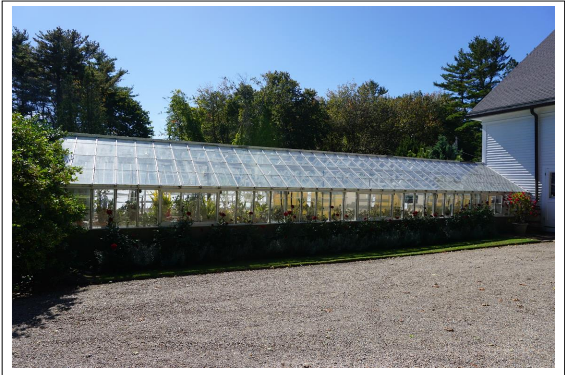
Photo # _201___ Description: Greenhouses, Fuller Gardens, 10 Willow Avenue Reference: WillowAve_10-2 Direction: Date taken: Sept. 2017
