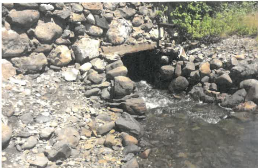
Philbrick Pond – Cobble weir. Outlet to Atlantic Ocean under Rt 1a.
