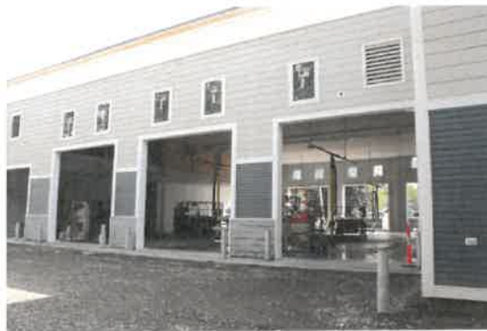
Thanks to David O'Brien for Pb. Safety bldg. photos
