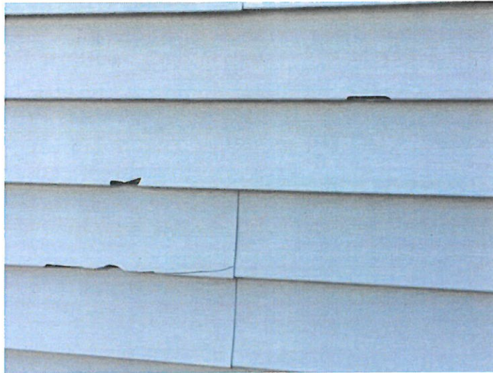
Siding damage - Town Offices / Police Building. Project to be completed in current FY2020
