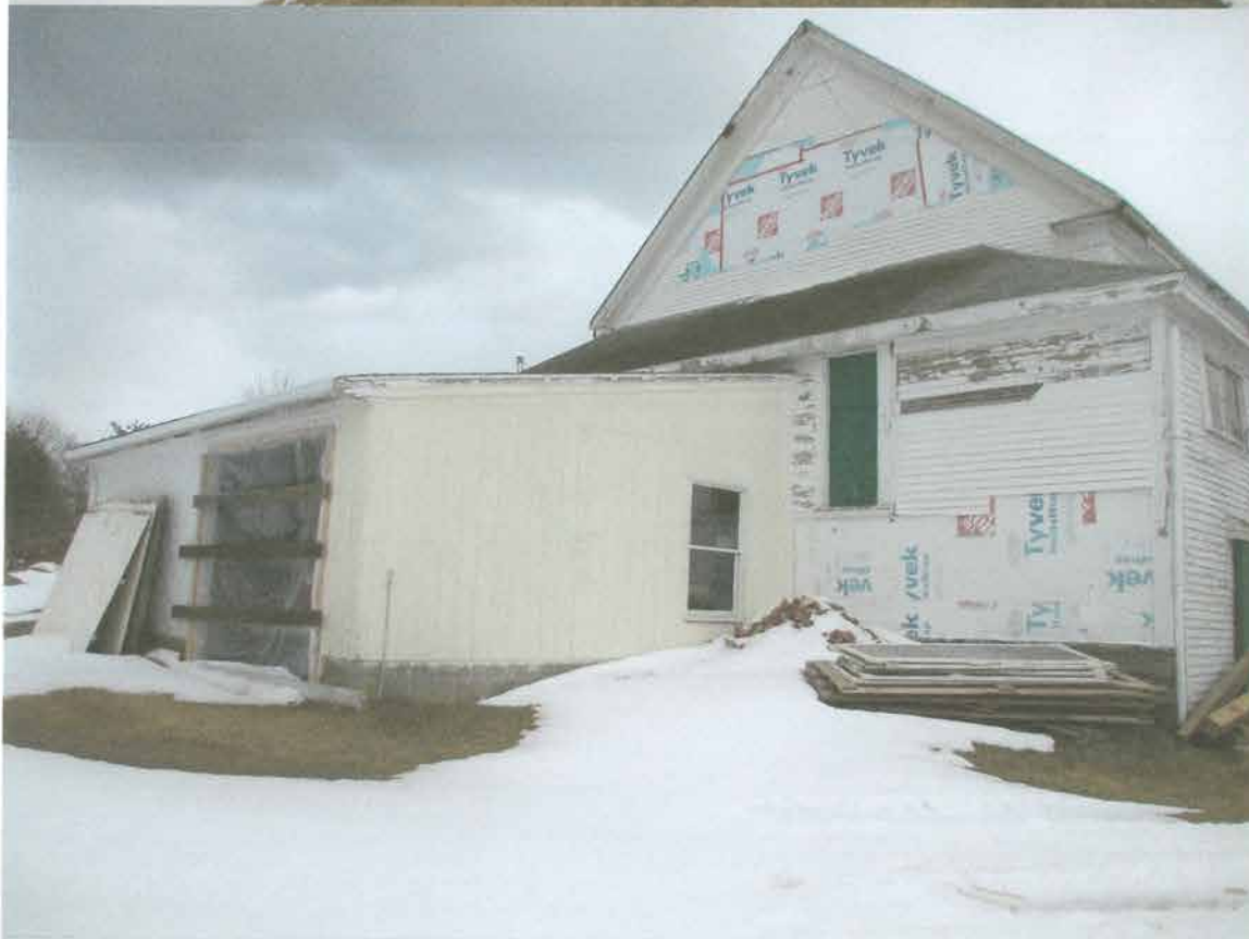
rear of main barn with lean-to
