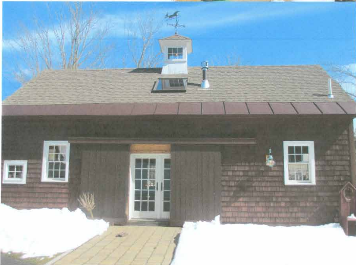
Rear with newer double door and sliding doors (not original)
