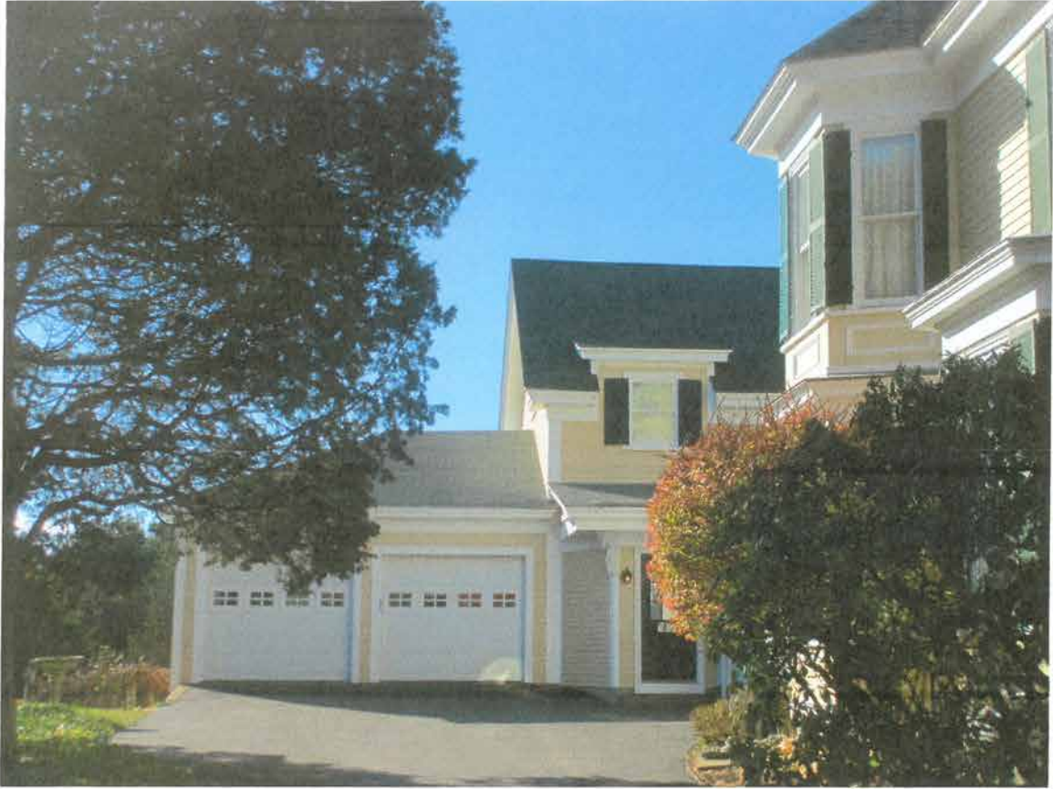
Right Side of Barn
