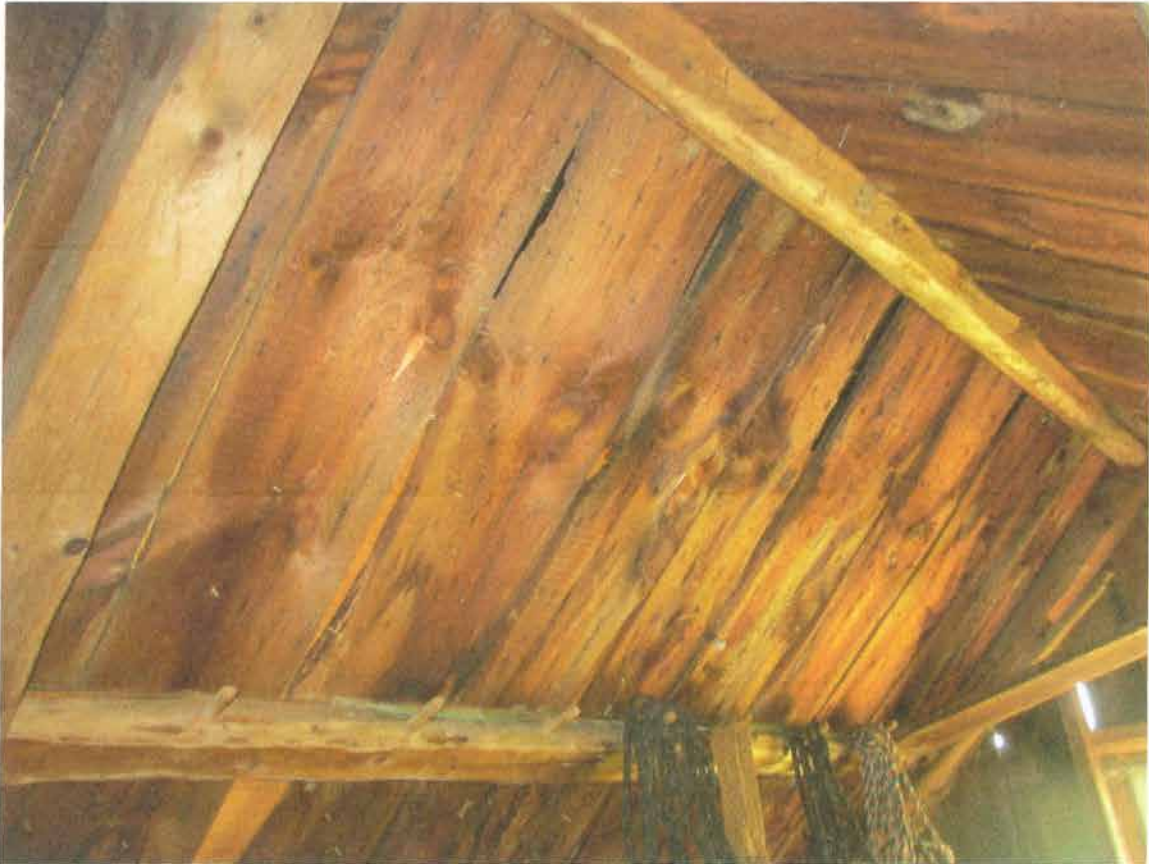
Barn / Workshop - Interior of Roof
