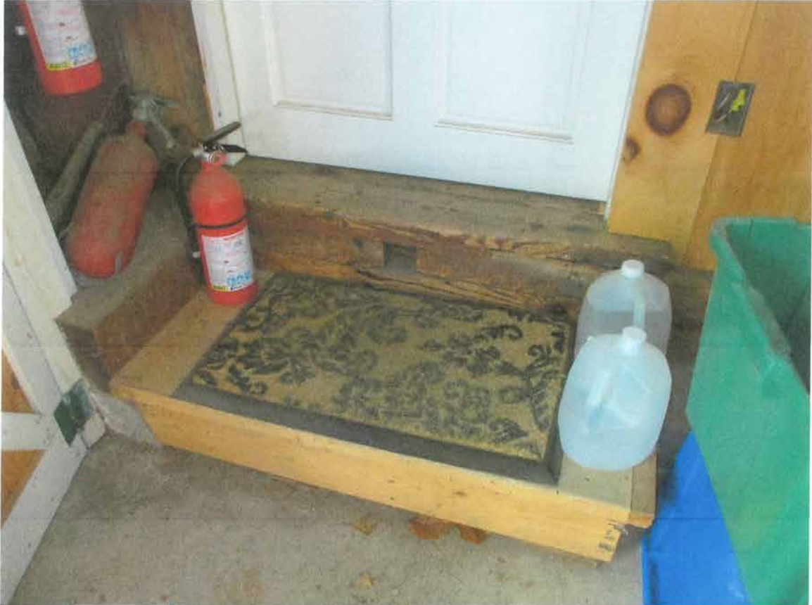
Original Barn Sill (just below door)
