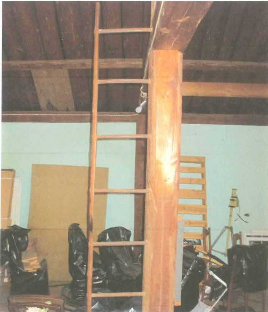
Hand Made Wooden Ladder in loft
