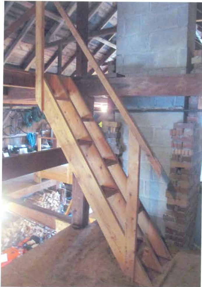
100 Mill Road Thomas Jefferson staircase
