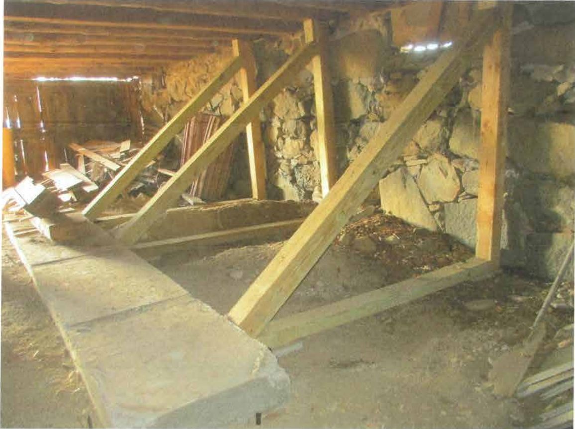
Reverse Buttress Against Western Side of Foundation
