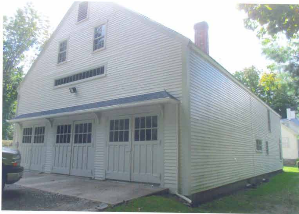
100 Mill Road - Rear + Left Side
