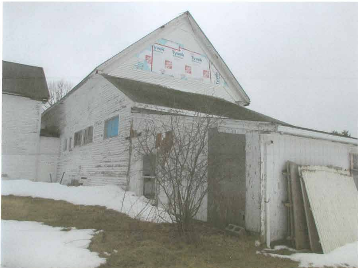
right side of main barn + lean-to addition
