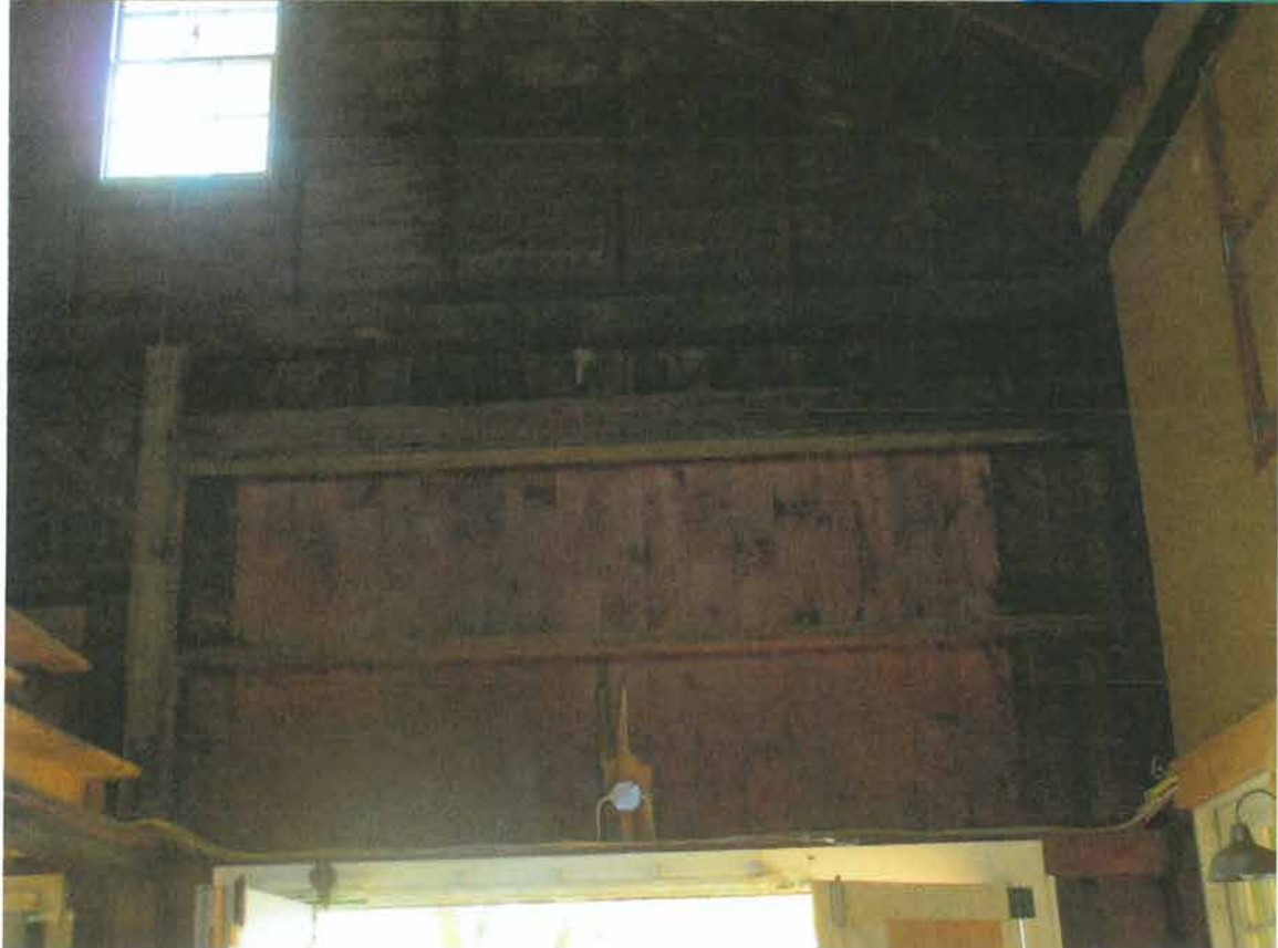
Original Header for Front Door
