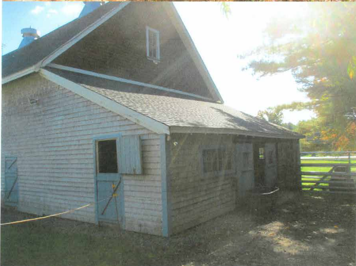
Rear Shed Addition
