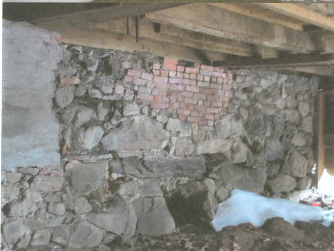
foundation under front of barn using bricks as fillers
