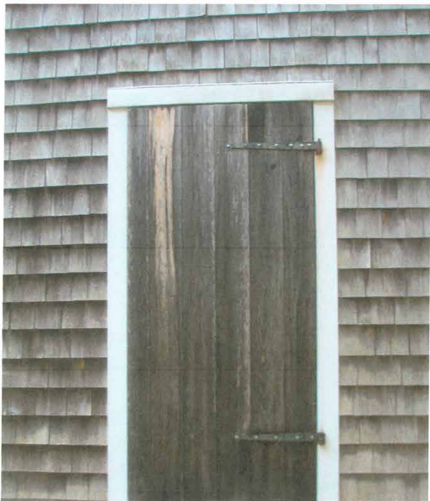
Back Door with Strap Hinges
