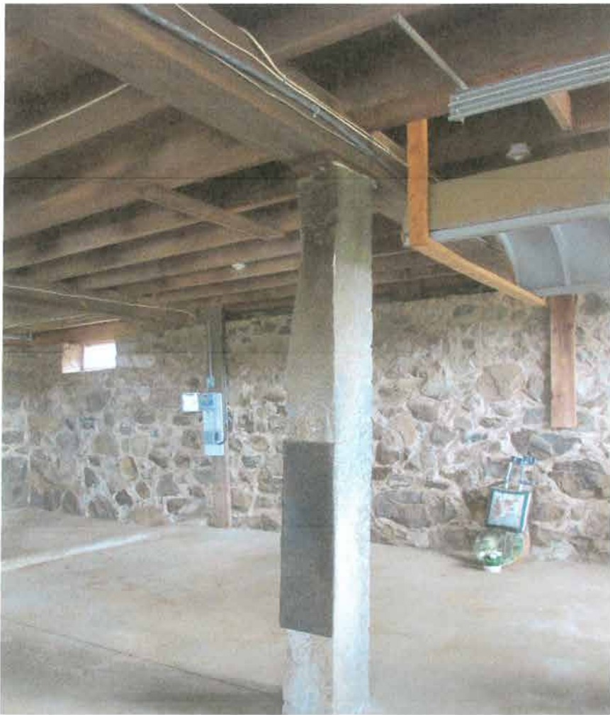
Cellar - Granite Support + Fieldstone / Cement Foundation
