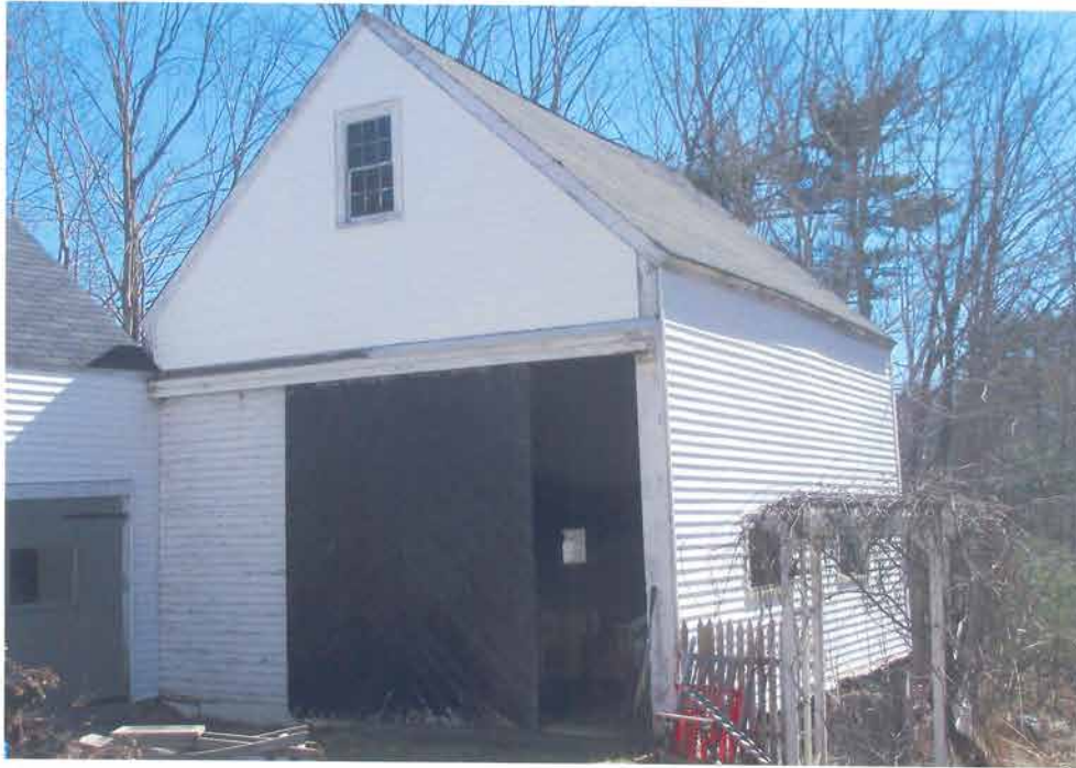
101 Mill Rd. - Front Facing West
