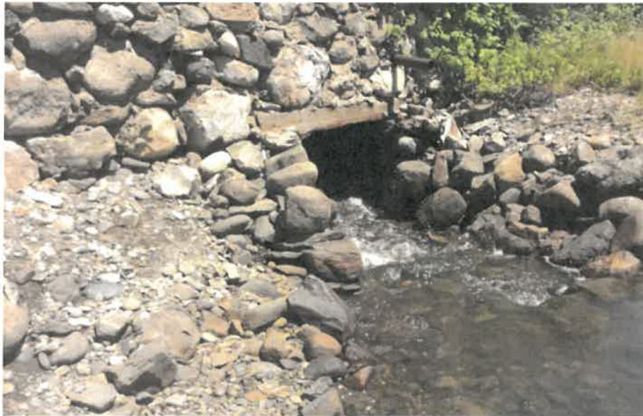
Philbrick Pond Cobble Weir outlet to the Atlantic Ocean under Route 1-A
