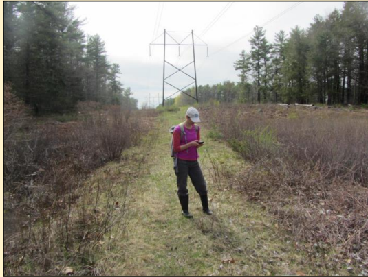
Wetlands D1 and D2. The pools are the result of a wetland being bisected by an access road within the powerline corridor.
