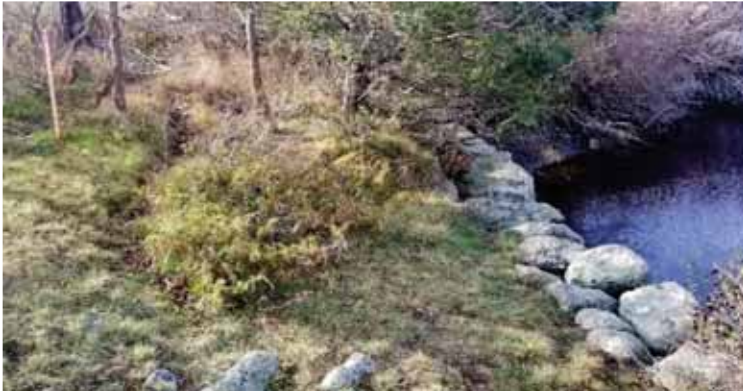
Figure 2 1900 Vintage Trolley Berm Surface
