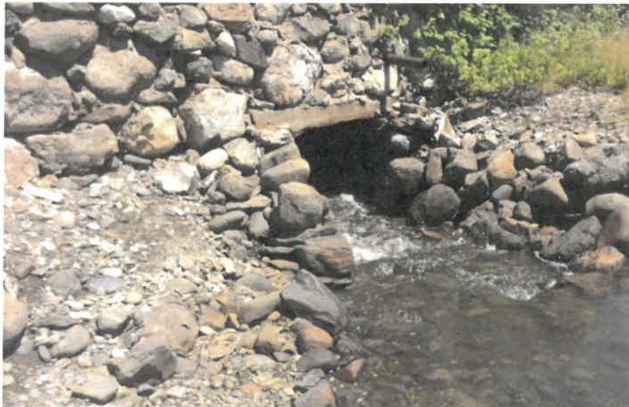
Philbrick Pond Cobble Weir outlet to the Atlantic Ocean under Route 1-A
