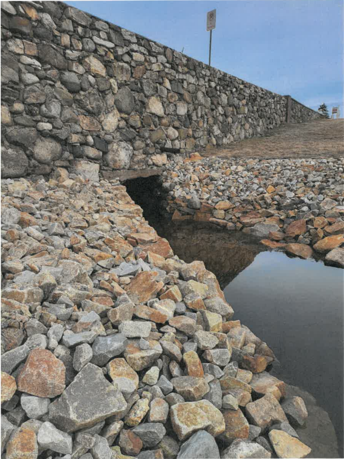
1. Philbrick Pond Culvert Inlet, March 15, 2022
