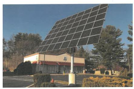
One, 24-panel Sun Action tracker using 385 kW bifacial panels & Sunny Boy Inverter. System size: 9.24 kW, with estimated annual production of 16,170 kWh
