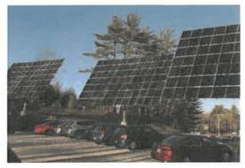
Three, 42-panel Sun Action trackers using 385 kW bifacial panels & Sunny Boy Inverter.
