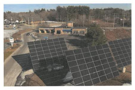
Three, 42-panel Sun Action trackers using 400 kW bifacial panels & Sunny Boy Inverter.
