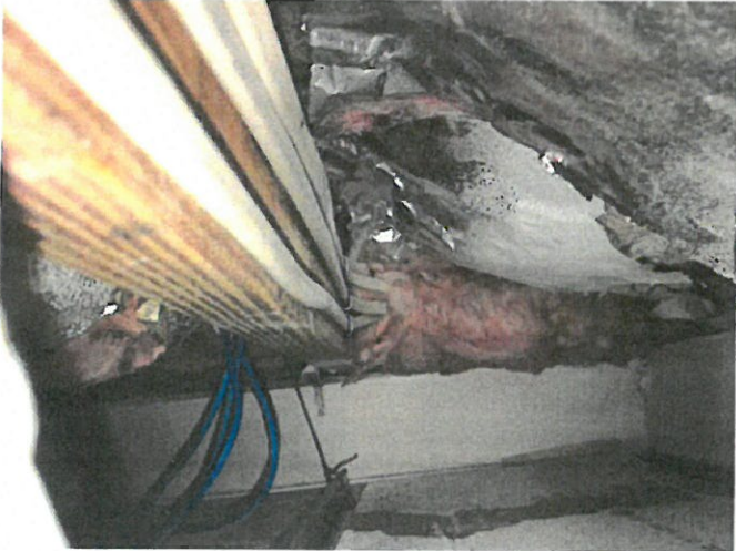
Figure 2 wall insulation shows to be uncompromised. Air sealing and sealed air chutes to be added in eve areas throughout.
