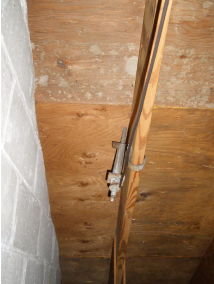
Photo 5: Antenna guy anchorage to truss top chord.
