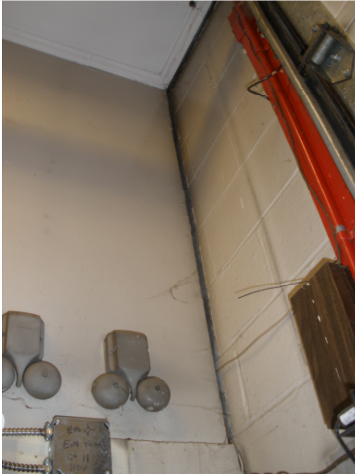
Photo 8: separation of south gable end wall (at right) from intersecting interior wall (left).
