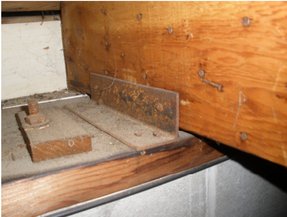
Photo 7: Truss bearing, clip angle, wall plate
