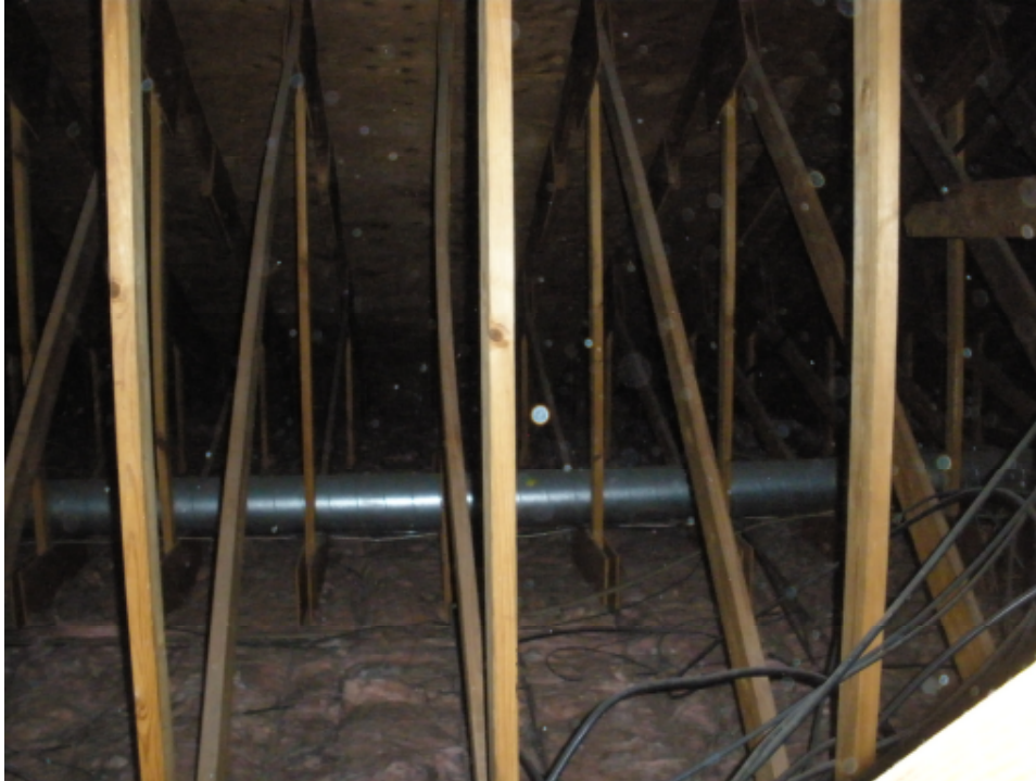
Photo 3: Bowed truss web diagonals, no thru-truss bracing.
