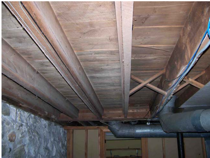
Tax Collectors Office Basement - Needs Insulation (Ceiling and FHA Ducts)
